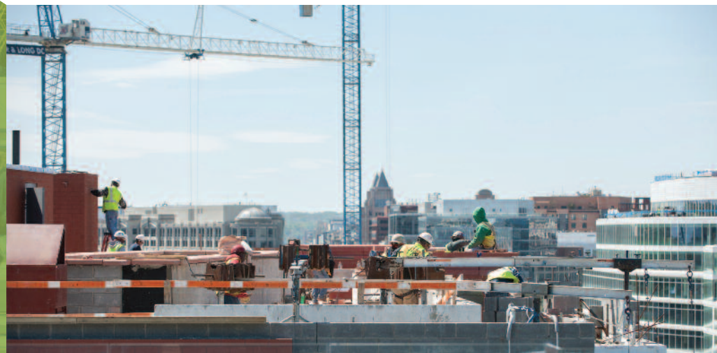
Construction at m.flats
