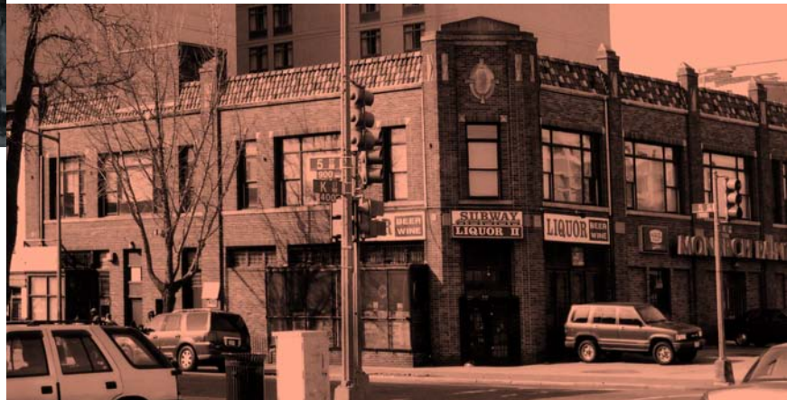
The Wittlin & Deckelbaum Building was built in 1932 to attract merchants to the 5th and K Street market after the closing of Center Market on Pennsylvania Avenue.
