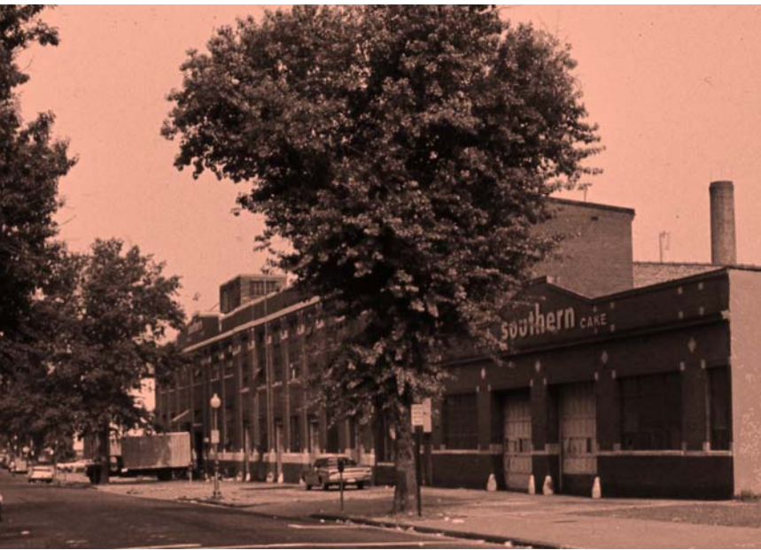
By the early 20th century, Schneider's Bakery, shown in this 1968 photograph, had expanded from Prather's Alley onto the 400 block of I Street, NW. (Courtesy Historical Society of Washington)
